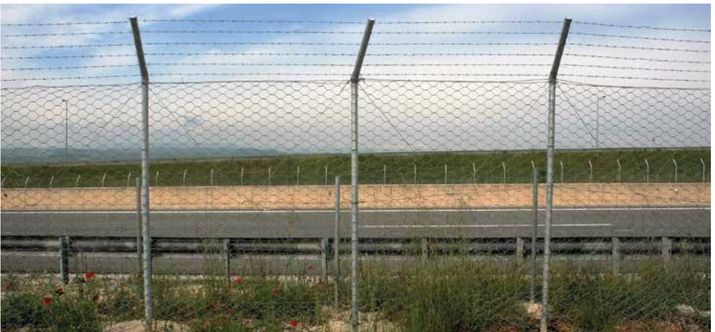
Fig. 10. Another view of the “bear-proof” reinforced fence, installed on the highway.
