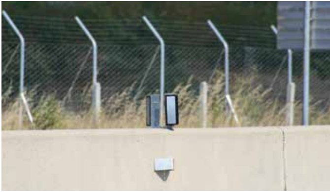
Fig. 4. WWR (Wildlife Warning Reflector) installed on the jersey of the highway.
