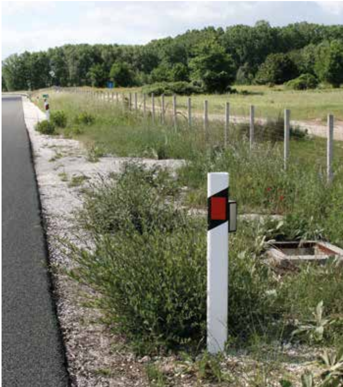
Fig. 5. WWR installed on delineator post of a county road.
