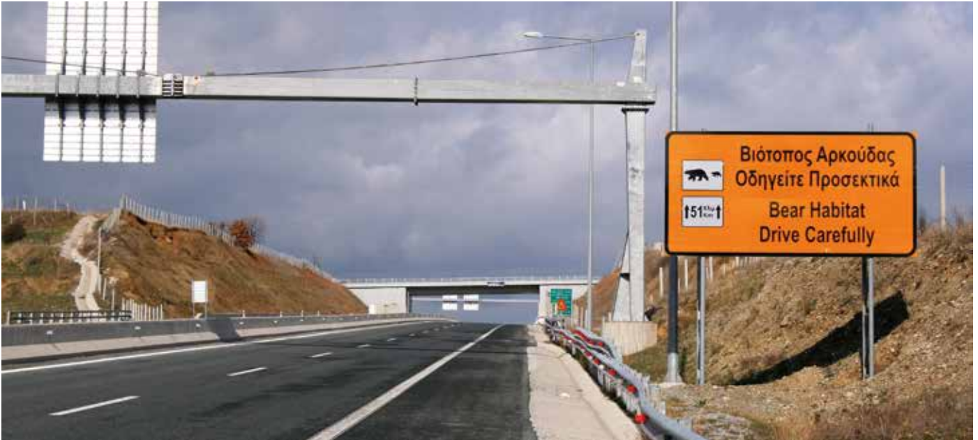
Fig. 8. Additional WRS installed on the KA45 highway by EGNATIA ODOS SA.
