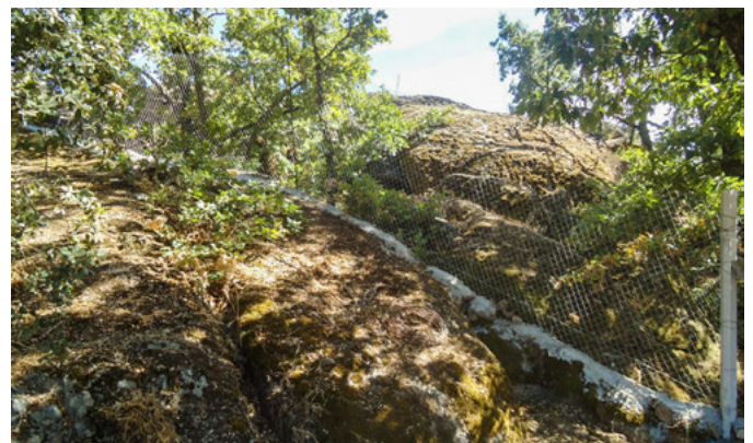
Fig. 7 Chain-link mesh fence at an ostrich farm with cement poles and concrete (masonry) base to prevent digging.
